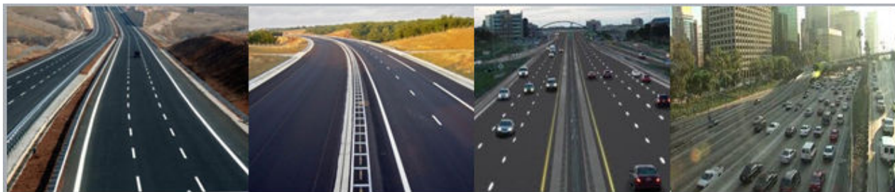
Figure 7: Dark colored roads and pavements absorb sunlight and emit in the far infrared.
